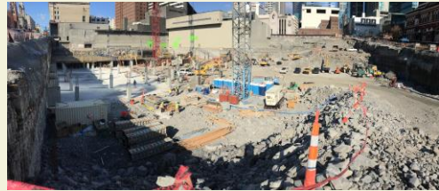
5 th + Broadway Parking Garage Level B2
