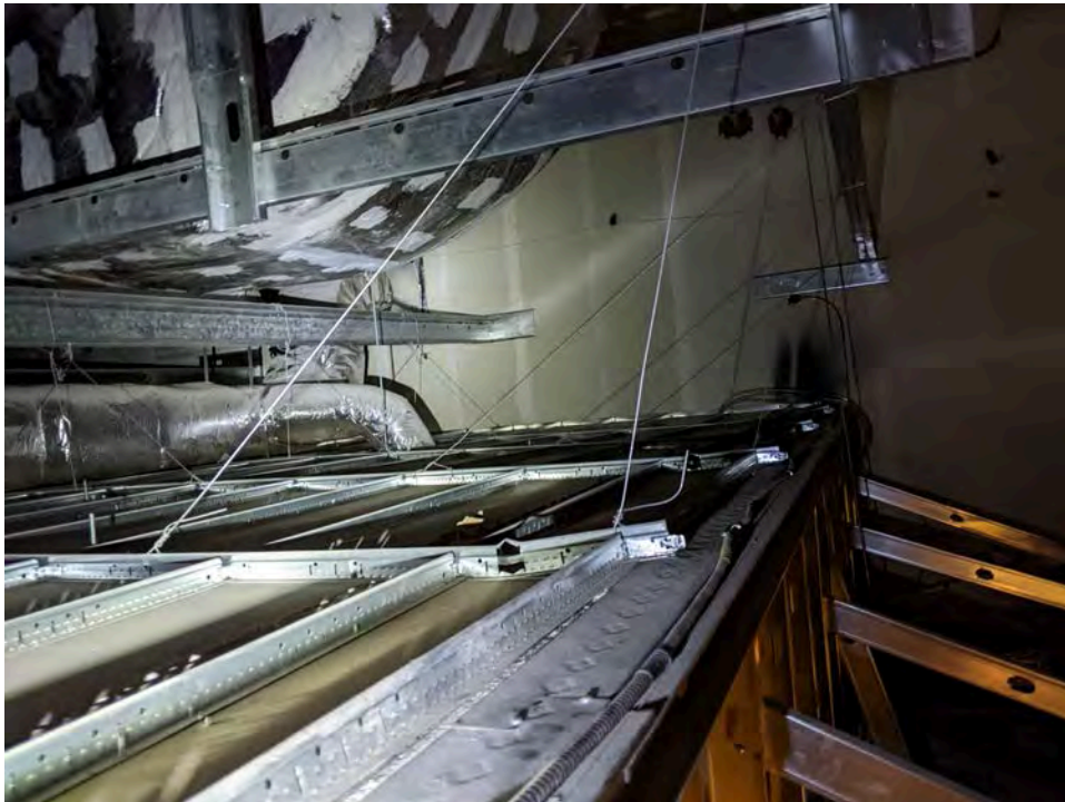
Photograph 6 – Sagging Ceiling Grid System
