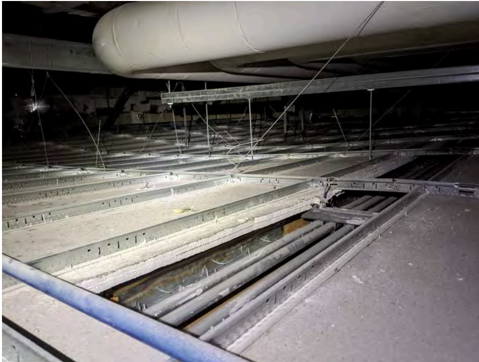
Photograph 7 – Sagging Ceiling Grid System
