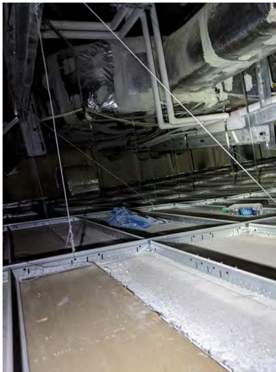
Photograph 4 – Sagging Ceiling Grid System
