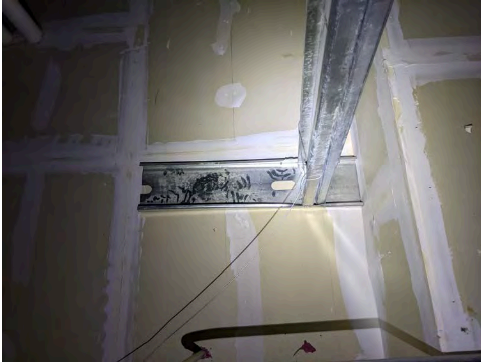
Photograph 9 – Rotated Light Gauge Support Framing
