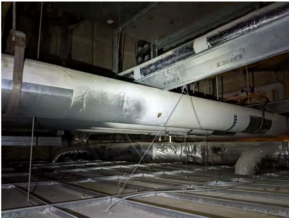
Photograph 8 – Light Gauge Support Framing Bearing on Piping
