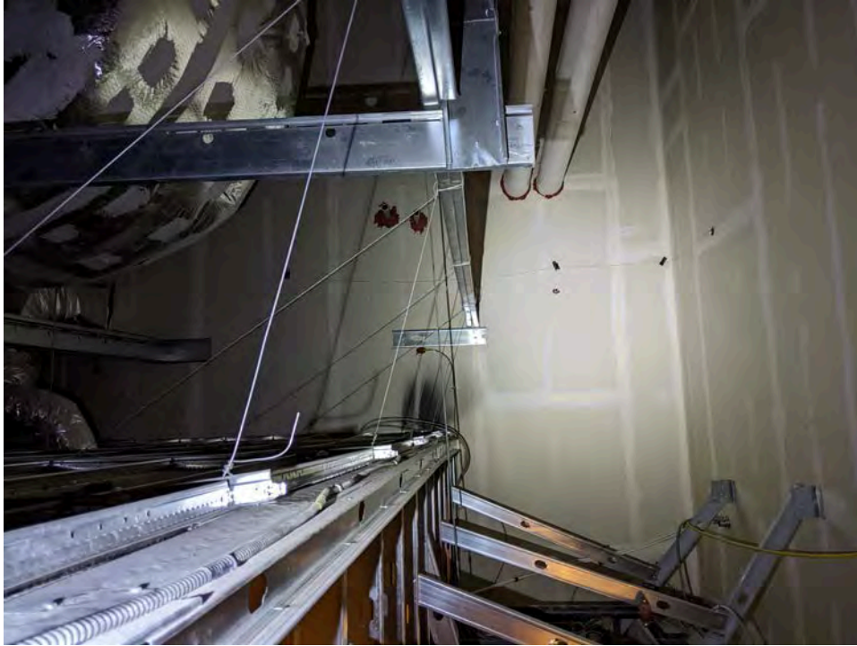
Photograph 5 – Sagging Ceiling Grid System
