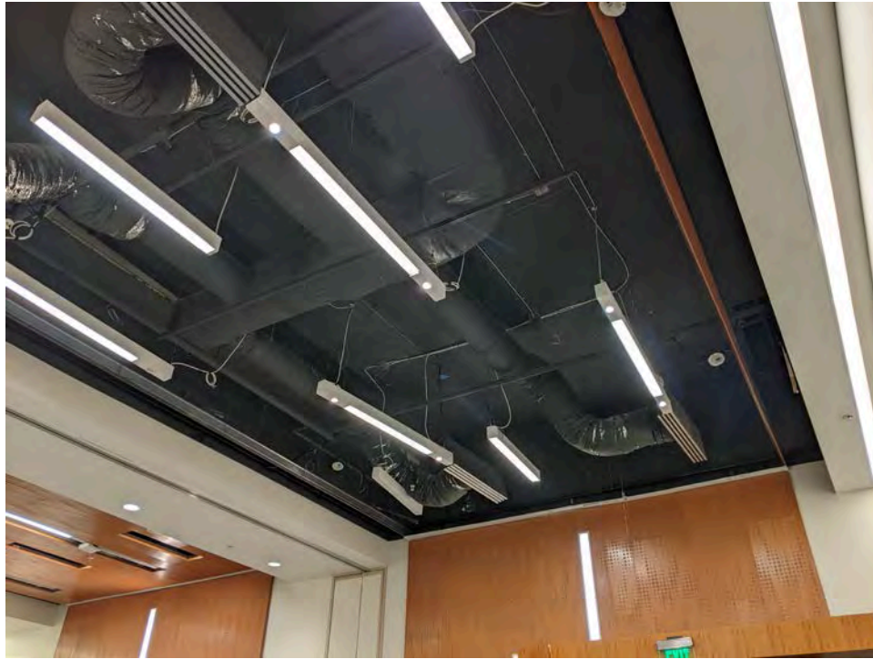
Photograph 1 – MEP above Architectural Ceiling
