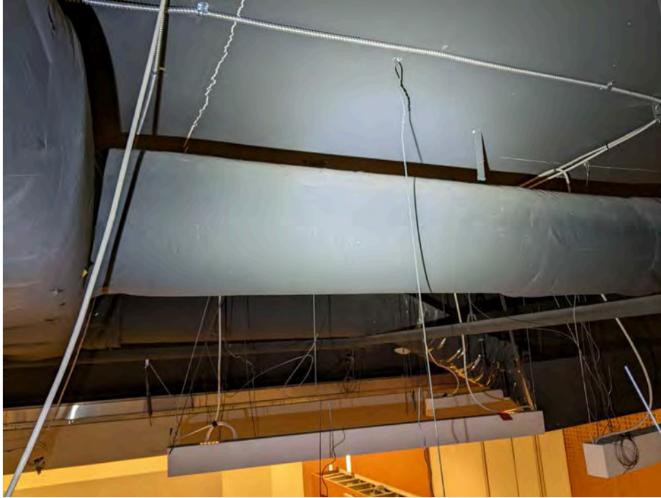
Photograph 3 – Gypsum Ceiling above MEP and Architectural Ceiling
