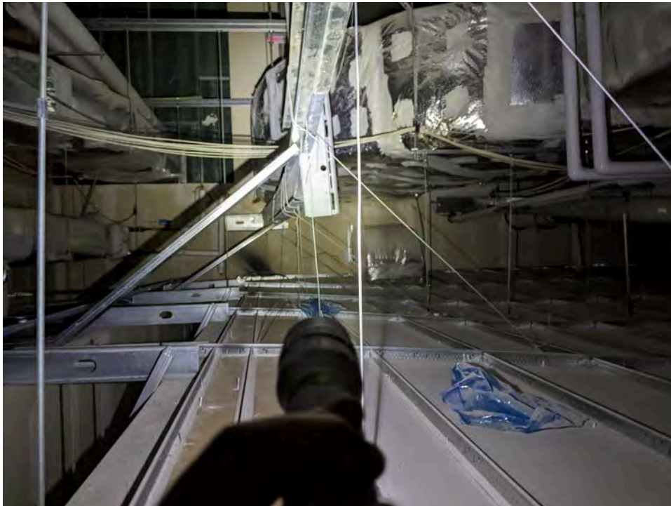
Photograph 10 – Bowing Light Gauge Support Framing
